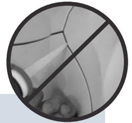
**Butt joint areas must not be glued or grouted.**
